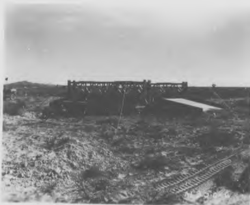
Before ↑ Bailey Bridge. Note: Loose ramp and broken walkway After ↓
